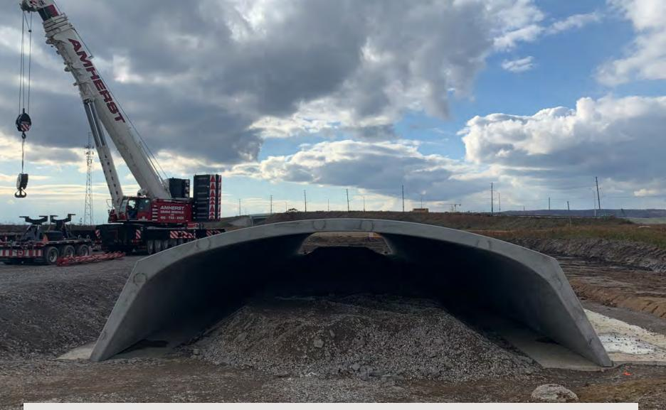
Arch culvert sections installed using large crane. Mixed gravel and stone material to be dispersed within the culvert to create natural substrate along Tributary A.
