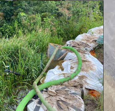
Flow isolation and fish basket in preparation for wing walls installation (July 24)
