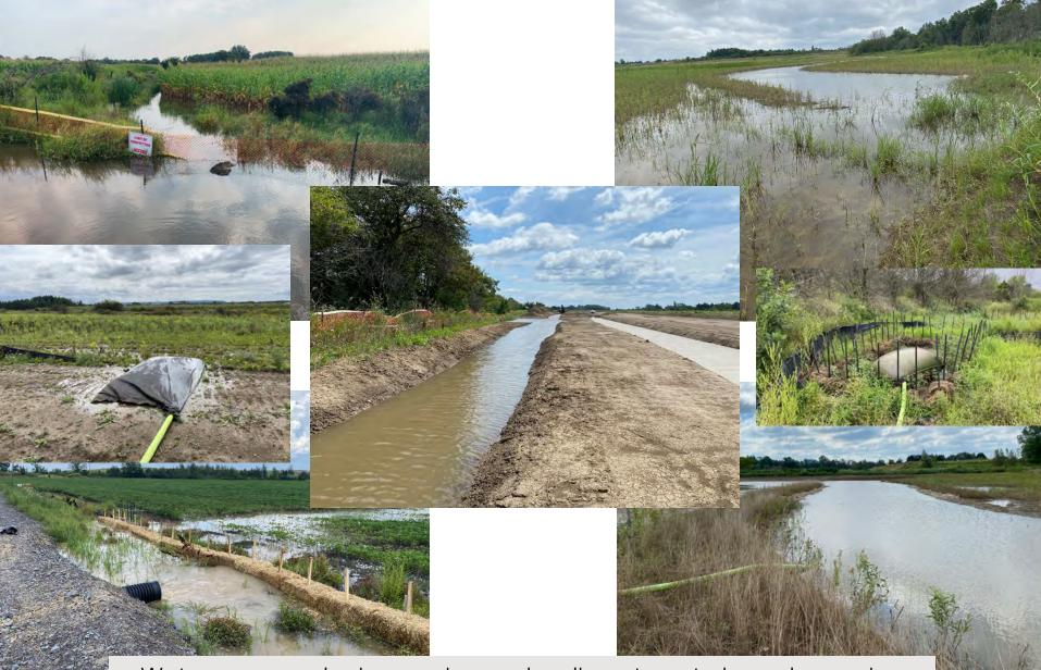
Water managed using erosion and sediment controls, and pumping
