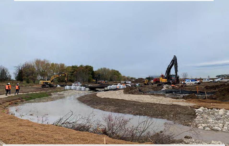
Natural channel design riffle-pool-riffle section now activated with flowing water. Deep water pools provide refuge and habitat diversity
