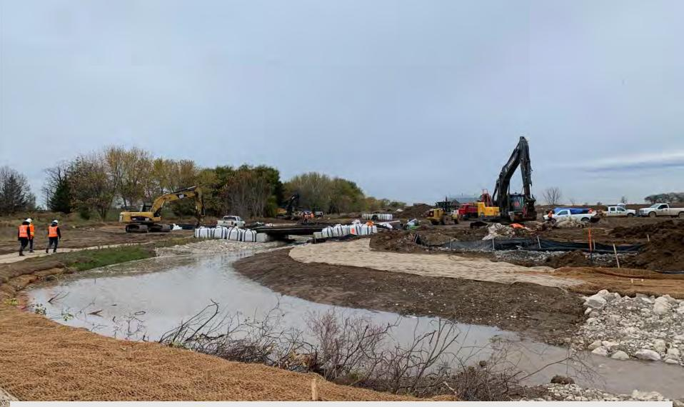
Natural channel design riffle-pool-riffle section now activated with flowing water. Deep water pools provide refuge and habitat diversity
