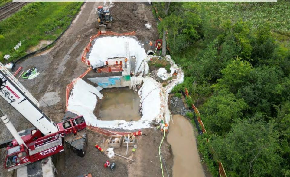
Additional isolation and dewatering of construction areas to install wing walls; Tributary A bi-pass pumping continues around coffer dams
