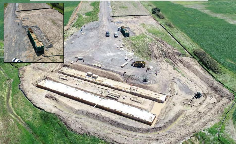
Isolation and containment of the construction area, with trenching, sumps, pumps and mobile treatment containment to manage dewatering
