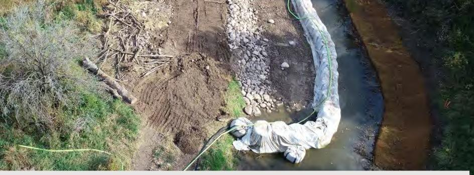
Matting and woody debris completed along new outer bank. Flows flipped to facilitate work on interior bank and riffle section prior to downstream connection
