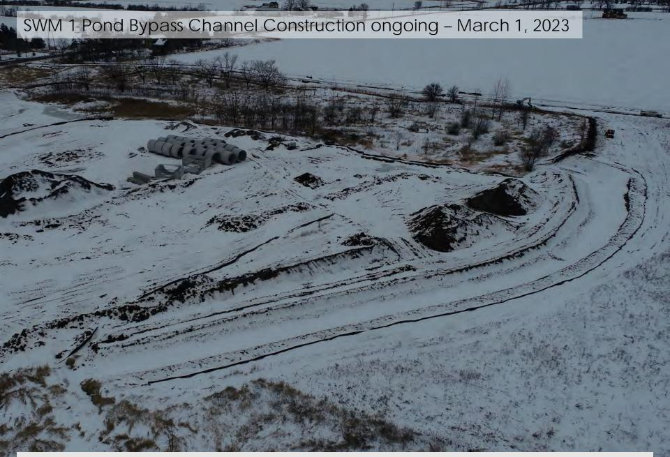
Temporary diversion channel constructed to accommodate construction of SWM Pond 1 to alleviate local flooding due to runoff from adjacent fields
