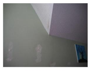
Plate 34: Patched plaster cracks in second floor laundry room of rear unit
