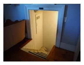
Plate 12: "Service" style back staircase descending view, also showing original pine floor and trim
