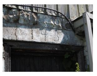
Plate 42: Cracked lintel above south entrance door
