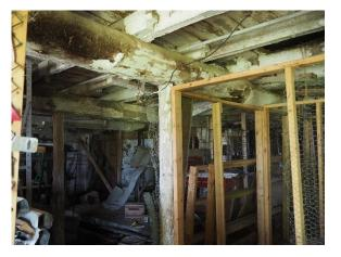
Plate 46: Interior split log and joists
