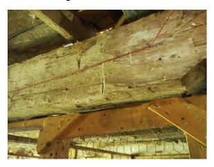
Plate 43: Hand hewn interior beams showing little damage
