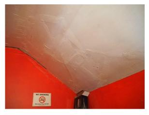
Plate 32: Patched cracked plaster on second floor bedroom of front unit
