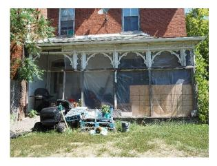
Plate 37: Peeling paint and missing support posts on front entrance porch
