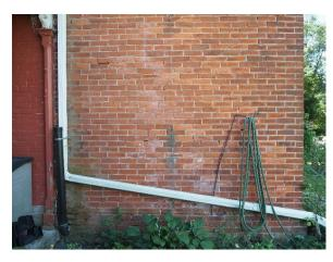
Plate 38: Efflorescence and missing mortar on west elevation near entrance porch
