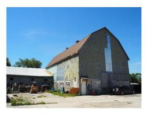
Plate 19: North and east façades showing gambrel roof and metal cladding, looking south
