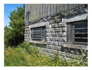
Plate 41: Rusticated concrete block foundation with limited cracking
