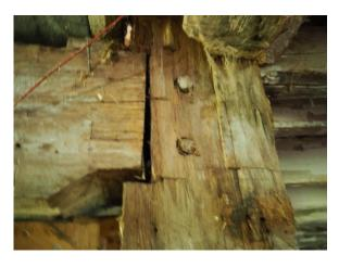
Plate 44: Mortise and tenon construction with some separation
