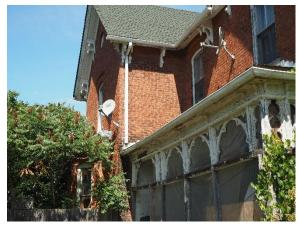
Plate 40: Disconnected downspout near front porch
