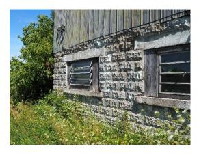
Plate 22: Rusticated concrete foundation, windows, and metal cladding on south façade, looking northwest
