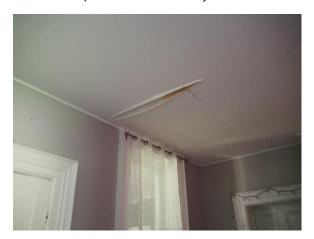
Plate 31: Peeling paint on ceiling of first floor front unit
