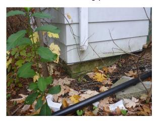
Plate 30: Downspouts draining to foundation
