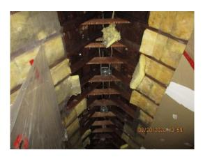
Plate 35: Water damage from roof leak
