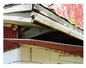
Plate 40: Collapsing exterior structural beams
