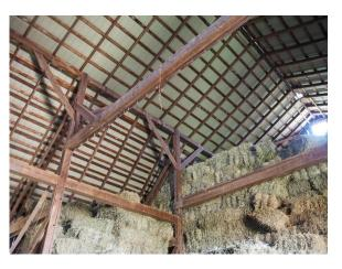
Plate 26: Machine cut beams, posts, and joists
