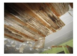
Plate 34: Water damaged ceiling tiles
