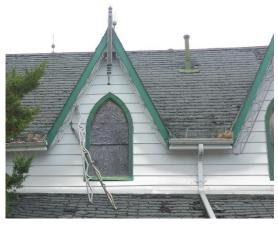
Plate 29: Worn paint and damaged bargeboard
