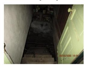
Plate 36: Basement stairs, considered unsafe for access
