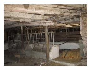
Plate 41: Interior structural beam of questionable integrity
