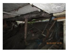
Plate 39: Collapsed foundation wall
