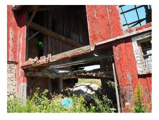
Plate 27: View of partially collapsed roof and hand hewn beams
