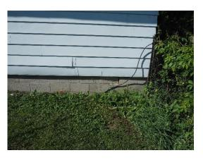
Plate 13: Settling and refilled cracks in the addition's foundation
