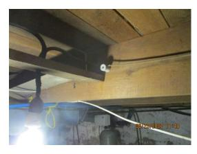
Plate 19: Active Knob and Tube wiring feeding light
