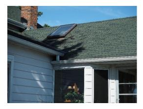
Plate 12: Localized areas of lifting shingles
