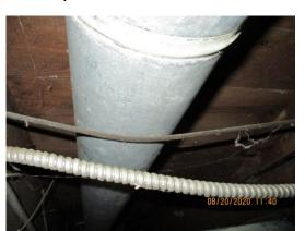
Plate 20: Knob and Tube wiring without protect from a forced air duct
