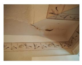
Plate 15: Water staining and cracking in second storey master bedroom
