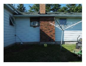
Plate 10: Gable addition, concrete block foundation and brick chimney on rear (northwest) façade, looking southwest
