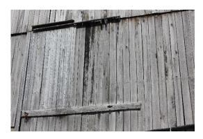
Plate 19: Sliding door and vertical timber cladding, southwest façade, looking north
