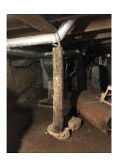
Plate 13: Timber support beams on concrete footing
