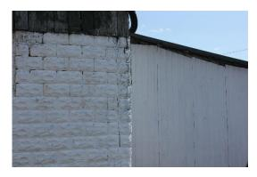
Plate 21: Rusticated concrete foundation and shed roof addition, looking east
