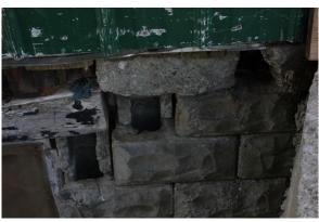
Plate 35: Broken blocks supporting rotting wooden lintels
