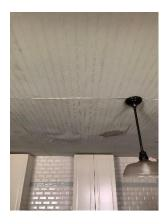
Plate 29: Water staining on kitchen ceiling from damage prior to roof repair
