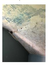
Plate 31: Cracking plaster on upstairs ceiling
