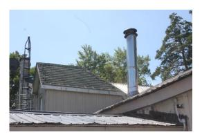
Plate 27: Shingled portions of roof in poor condition, looking southwest
