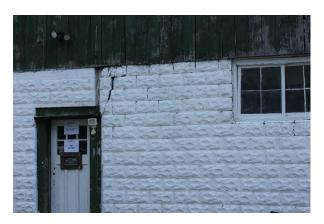
Plate 34: Localized cracking in the concrete foundation of the barn, looking west
