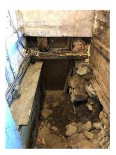
Plate 32: Cracking plaster, foundation shift and stairway obstruction on the basement staircase
