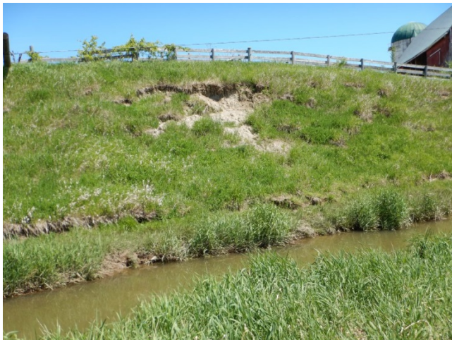
Photo 54: Upstream of Transect 9; slumping on creek bank.
