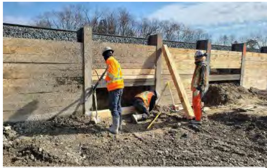
LBL West – Lagging work & Anchor Testing (February 15 to March 1, 2024)
