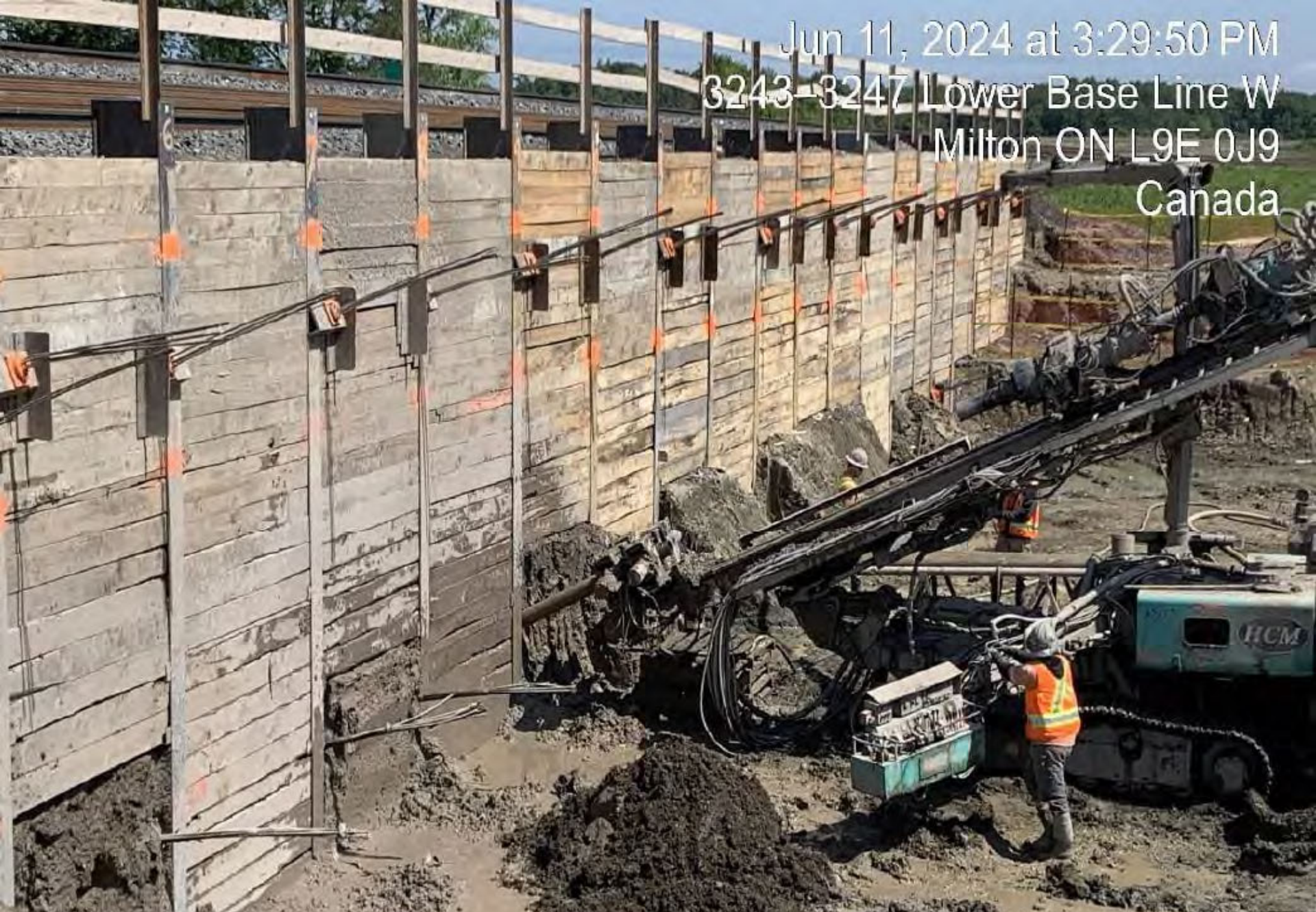
Lower Base Line W lower-level tie back installation - June 11, 2024
