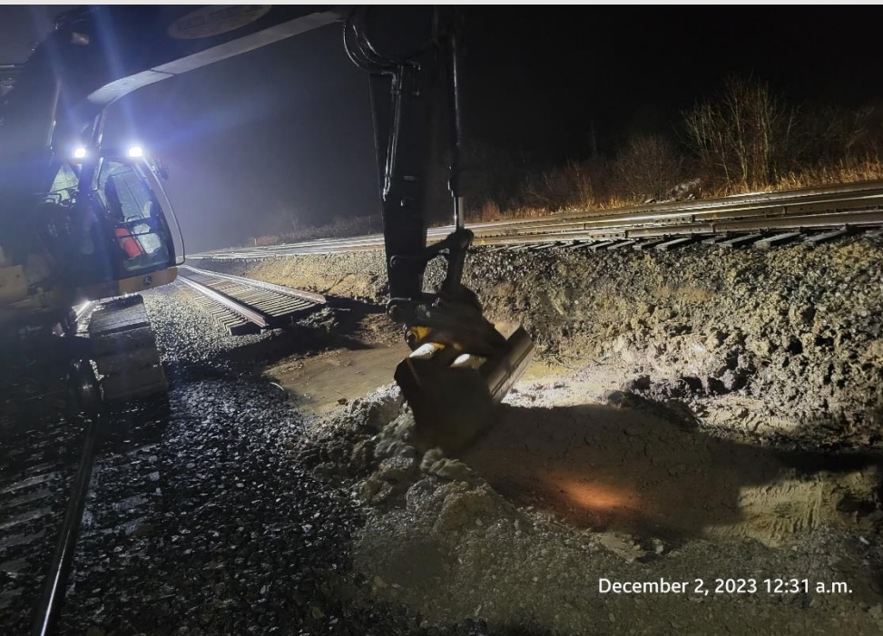
Sub-excavation works
