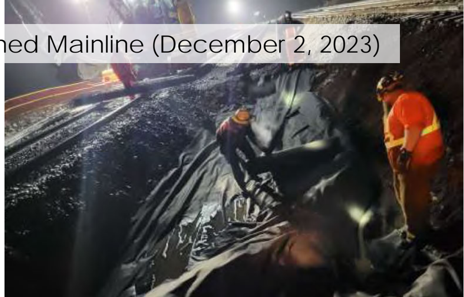
Installation of geo-textile and geo-grid
