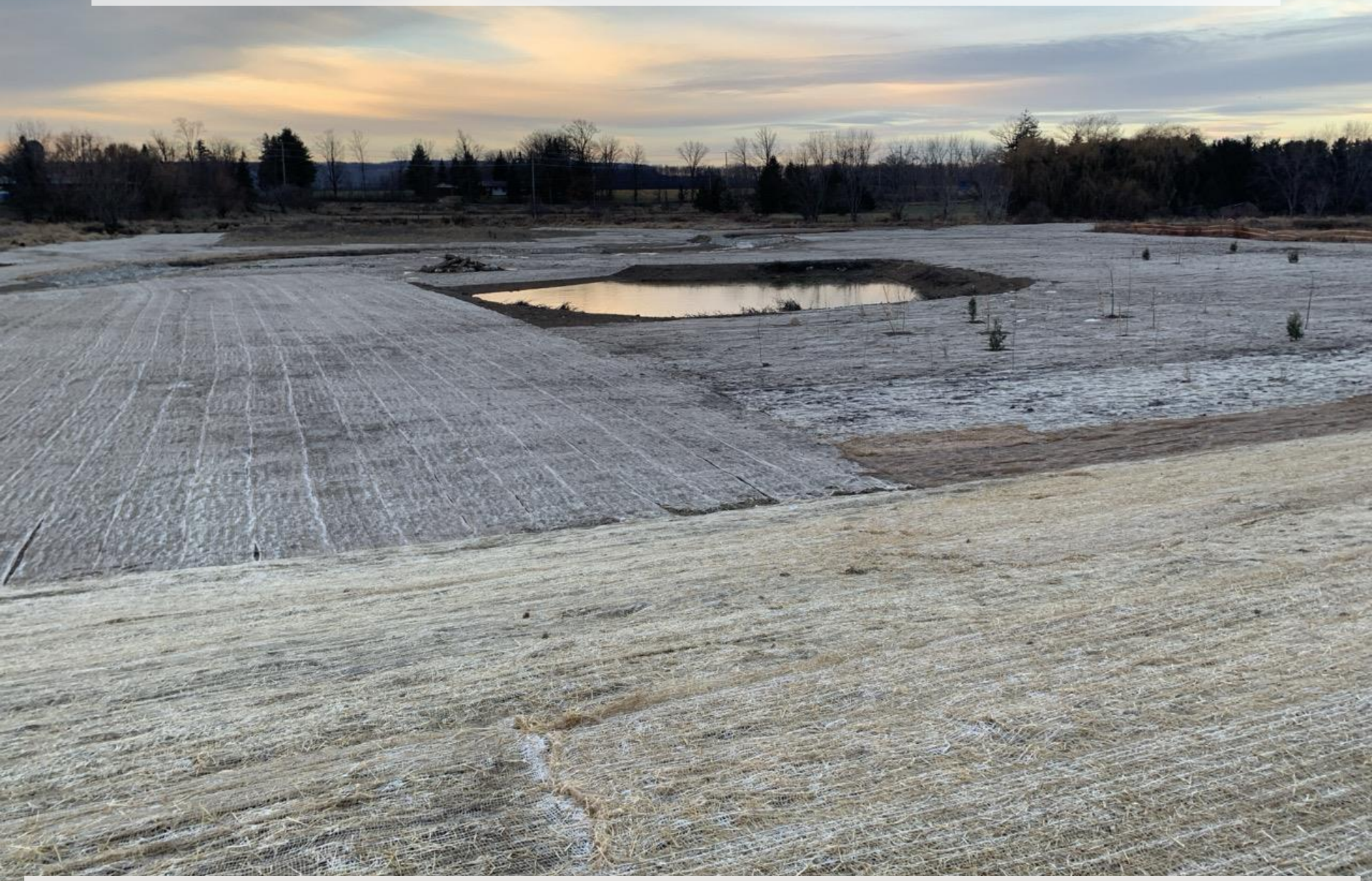
Matting installed on Indian Creek Valley slope (former location of access ramp)
