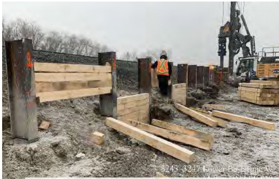
LBL West – Lagging work & Anchor Testing (February 15 to March 1, 2024)
