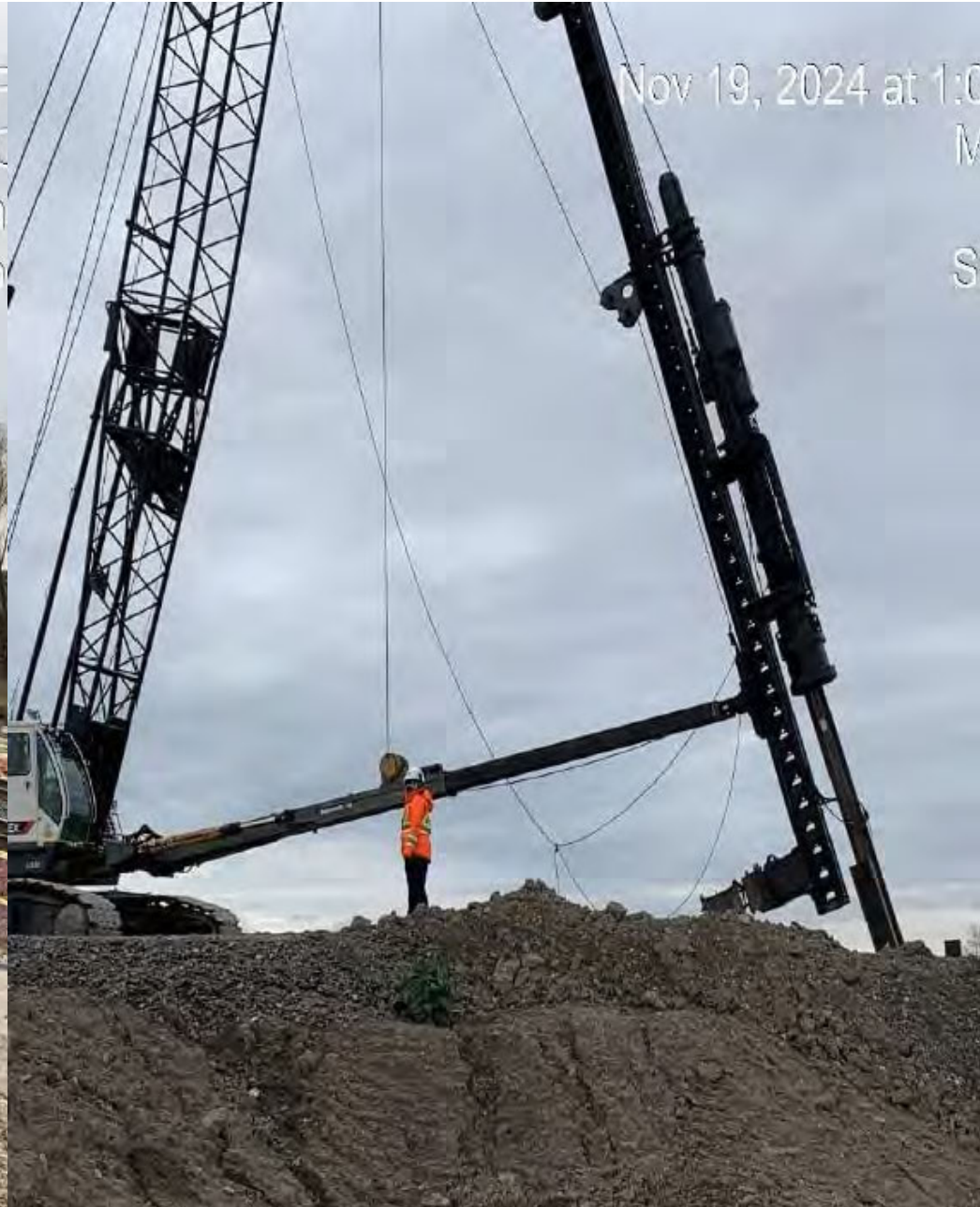
H-pile driving at east abutment – Nov. 19, 2024
