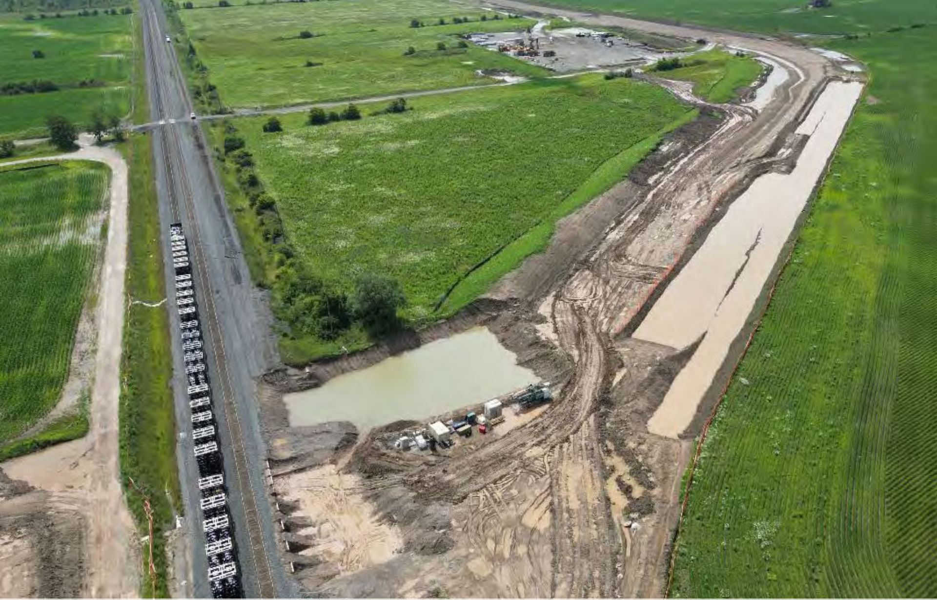
Britannia Access Rd – Ongoing excavation of west ditch and grade separation for crane pad (June/July 2024). Impacted by heavy rainfall week of July 8 & 15 and required water pumping/removal.
