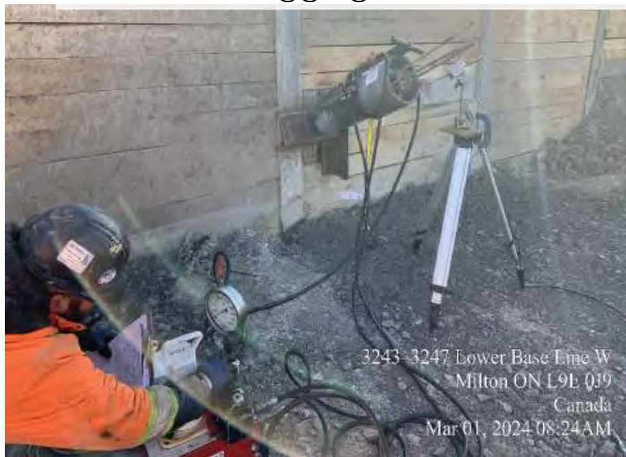
LBL West – Lagging work & Anchor Testing (February 15 to March 1, 2024)
