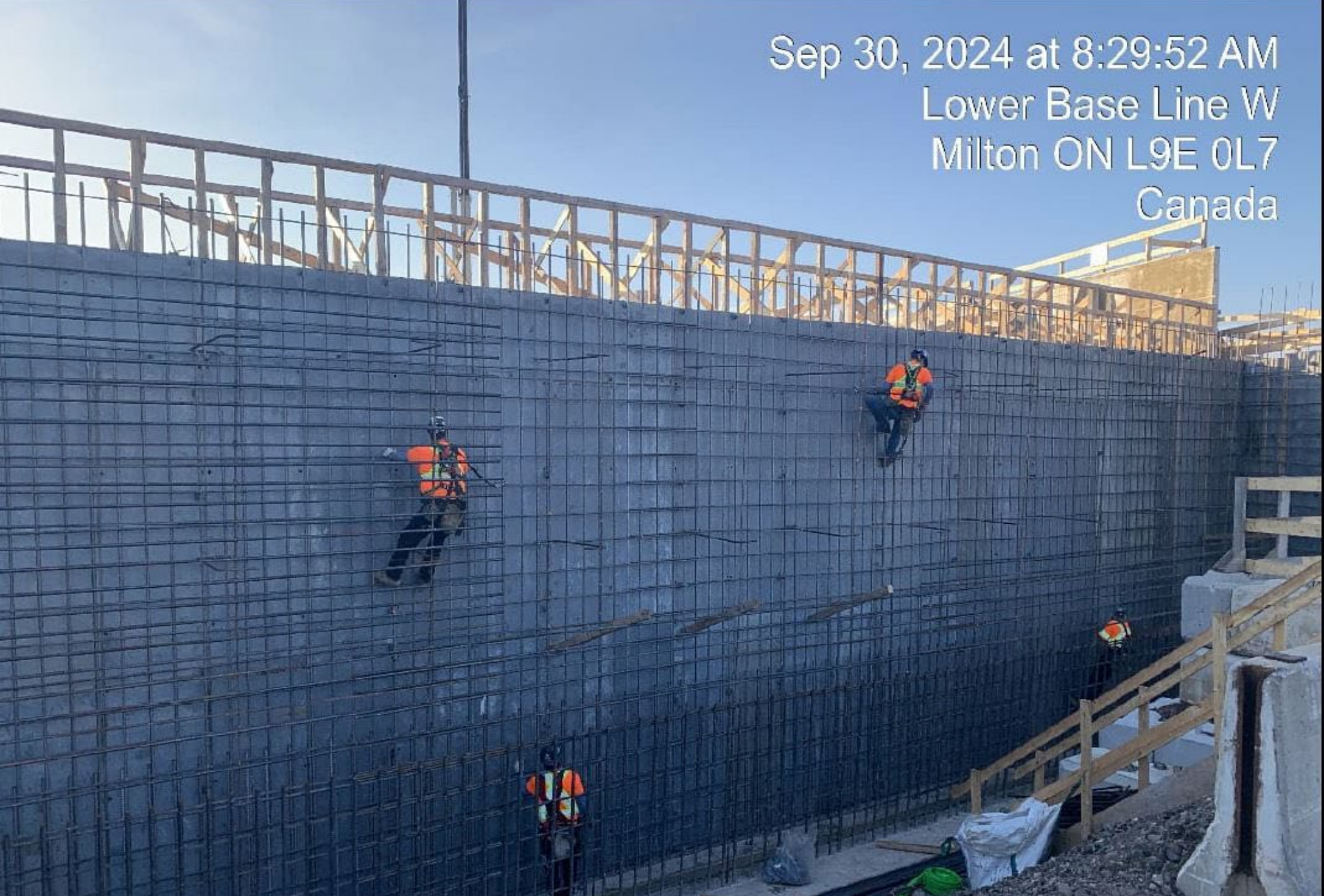
LBL Bridge – Installation of rebar steel for north abutment east wing wall Sept 30, 2024
