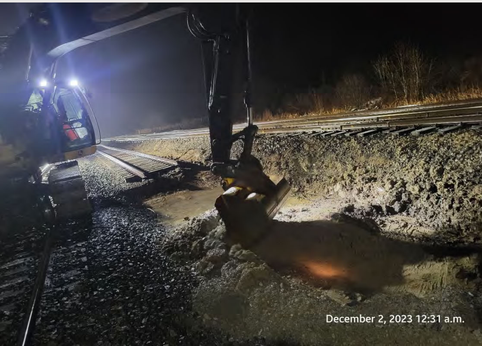
Sub-excavation works
