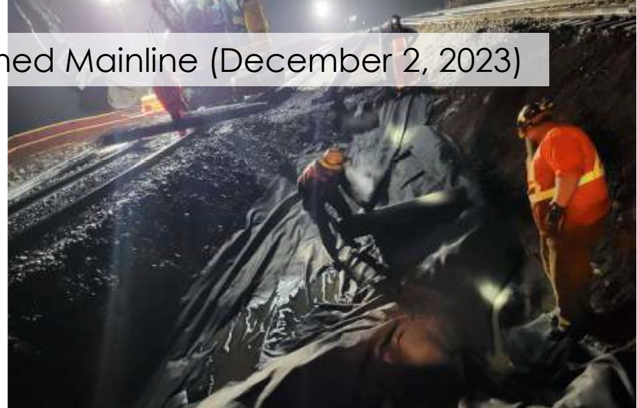
Installation of geo-textile and geo-grid
