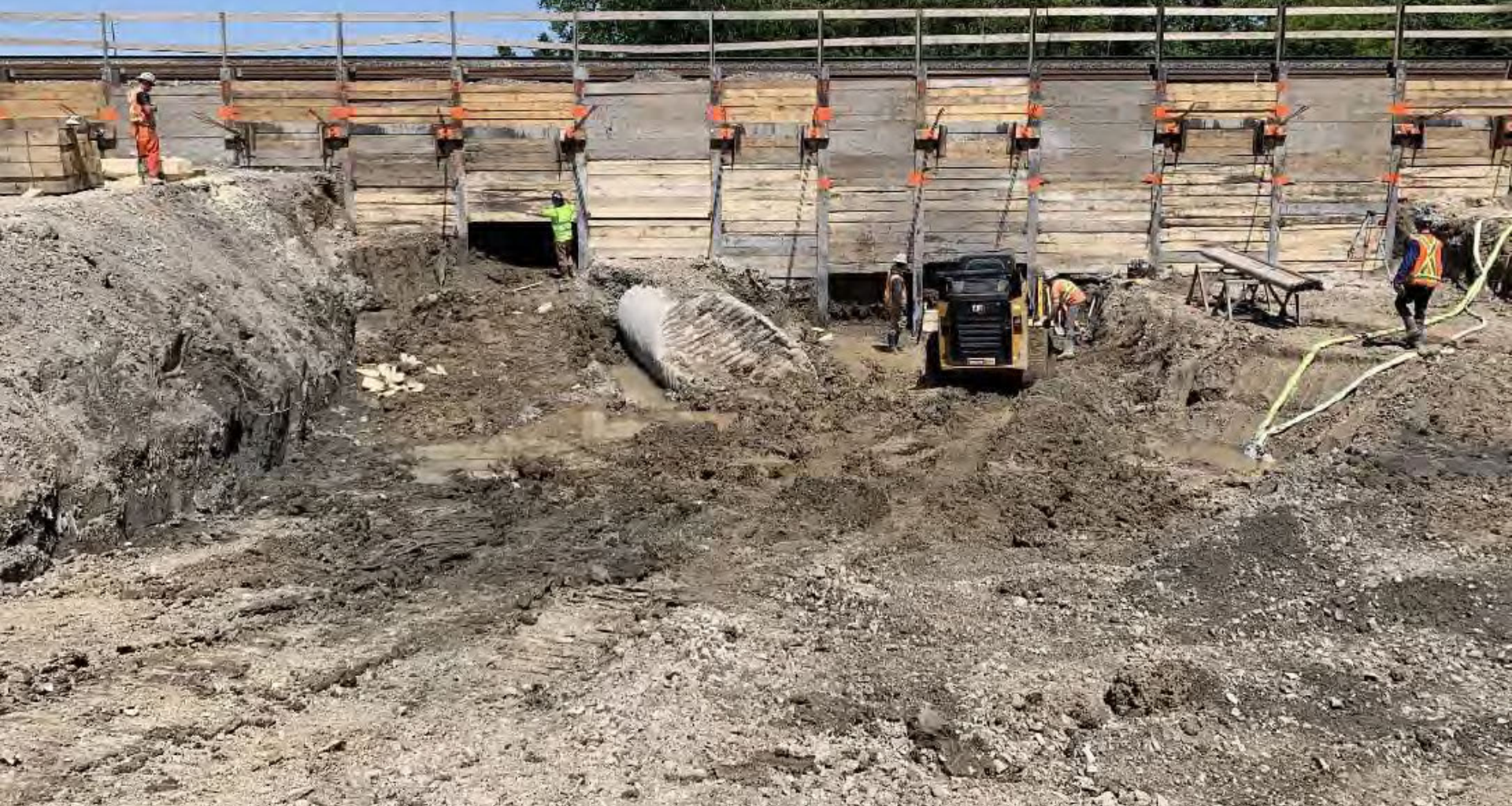
Lower Base Line W excavation and continued wood lagging install – May 30, 2024
