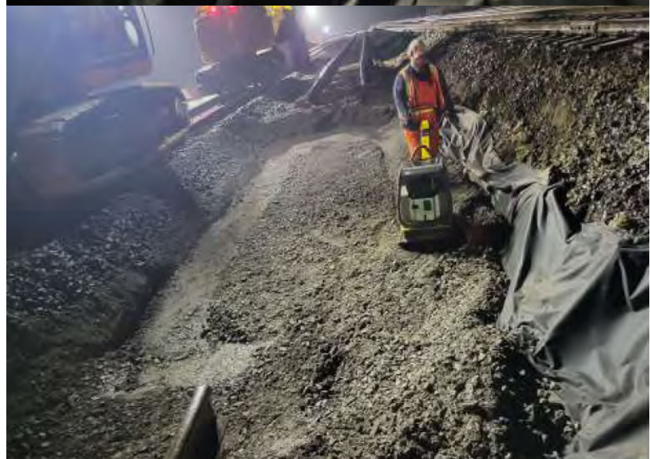
Compaction with tamper plate
