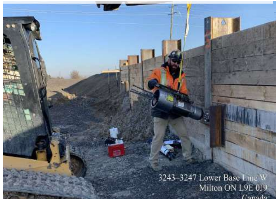
LBL West – Lagging work & Anchor Testing (February 15 to March 1, 2024)
