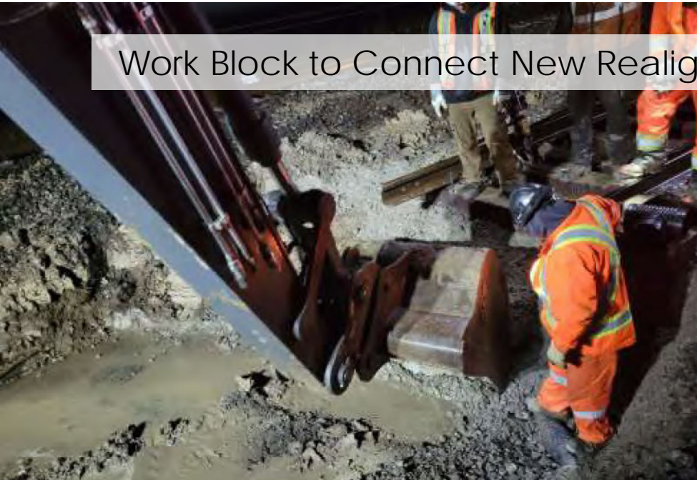
Sub-excavation works
