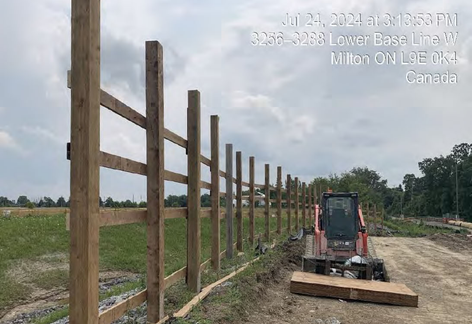
Lower Base Line Road – Hoarding noise wall Installation commenced July 24, 2024
