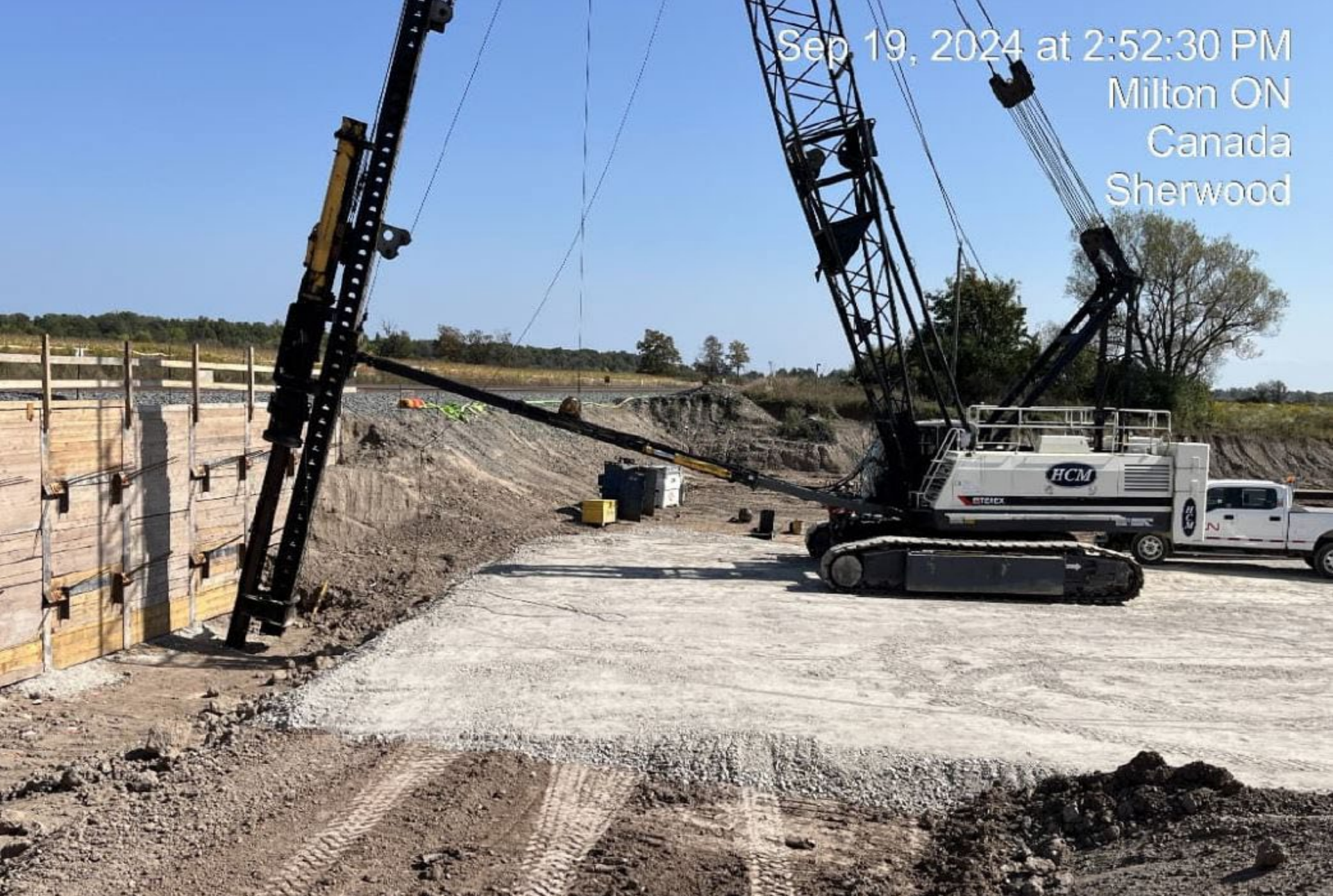
Britannia Access Rd Bridge – Begin pile driving along west side of bridge - Sept 19, 2024
