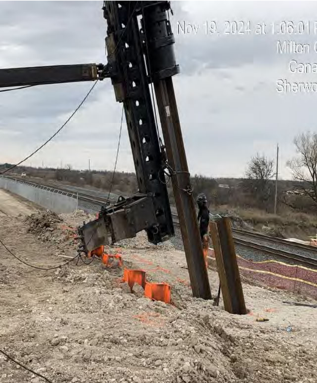
H-pile driving at east abutment – Nov. 19, 2024
