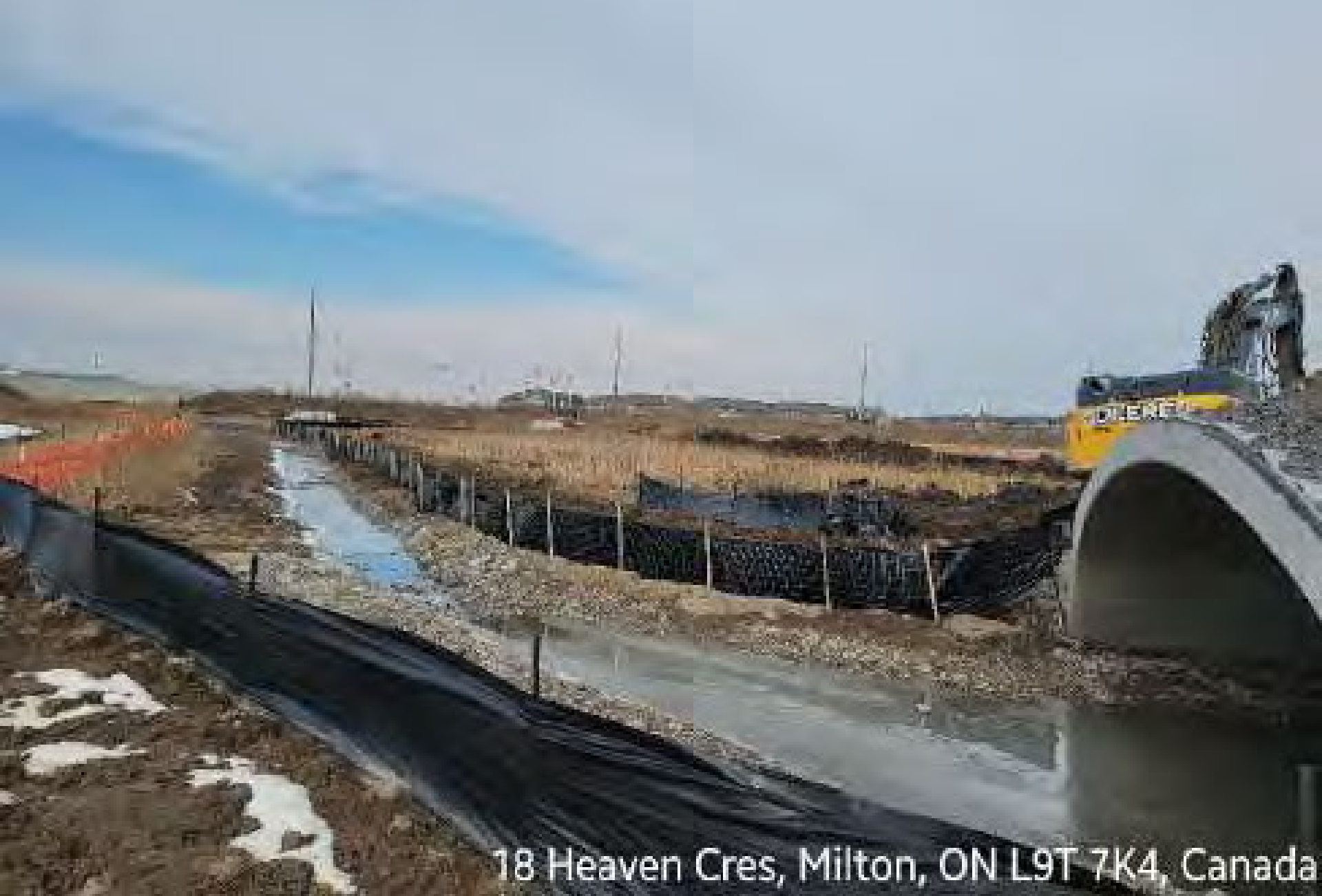
Britannia Road – Relocated silt fence at inlet of Culvert 1 (Feb. 21, 2024)
