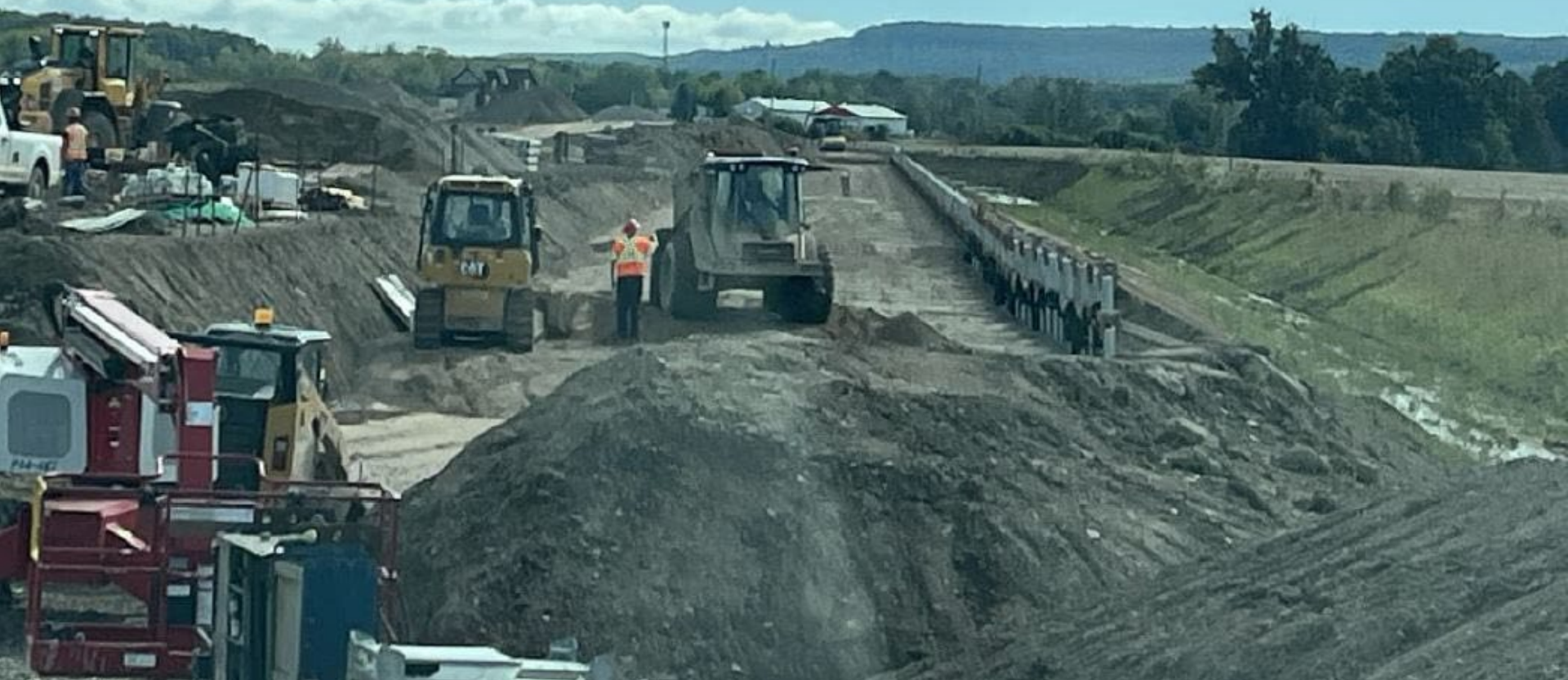
Britannia Access Rd – Backfilling of material along west RSS wall – Sept. 27, 2024
