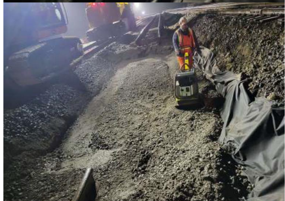
Compaction with tamper plate
