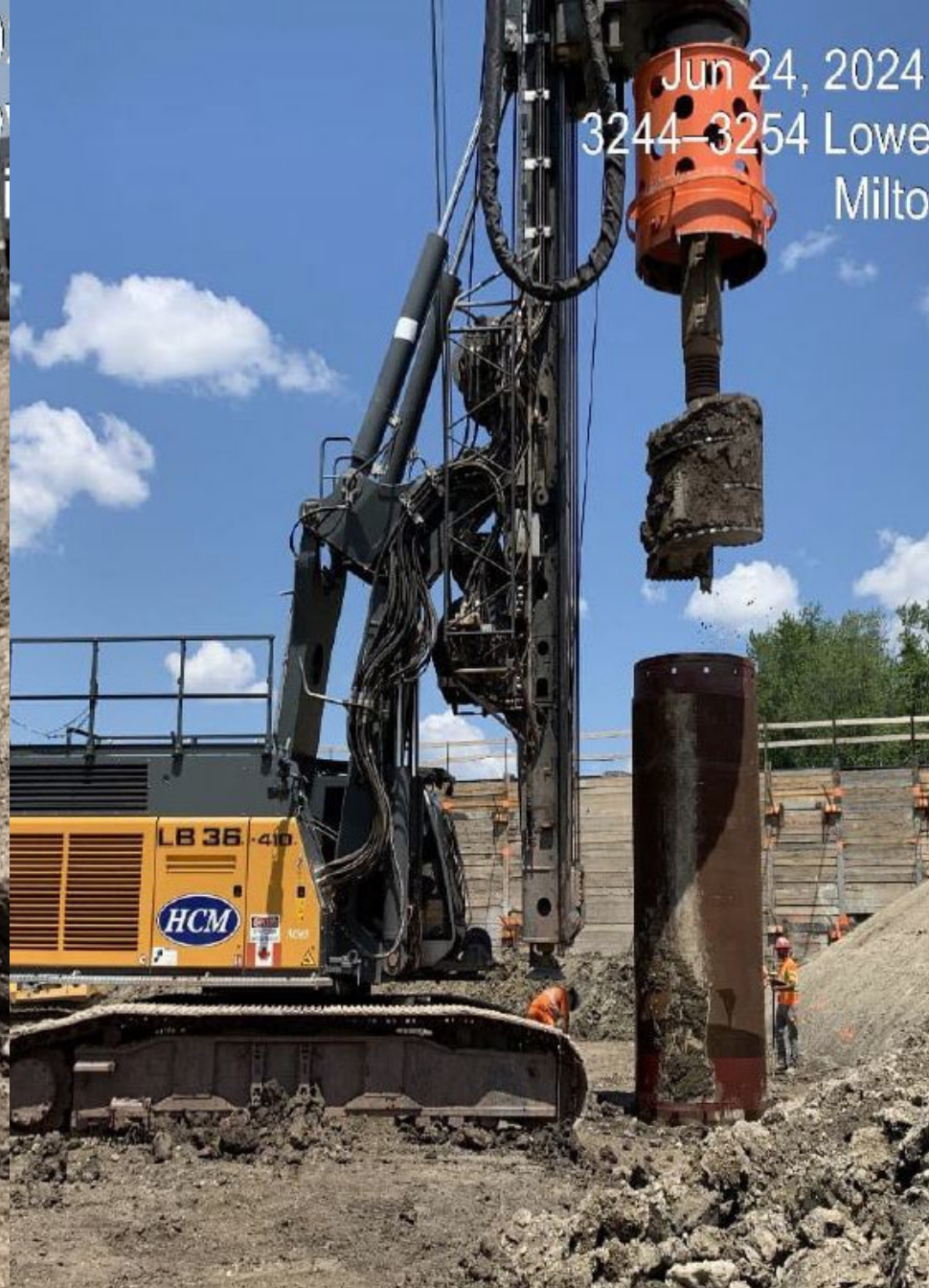
LBL West – Drilling prep and caisson installation for crane pad June 24- July 2, 2024
