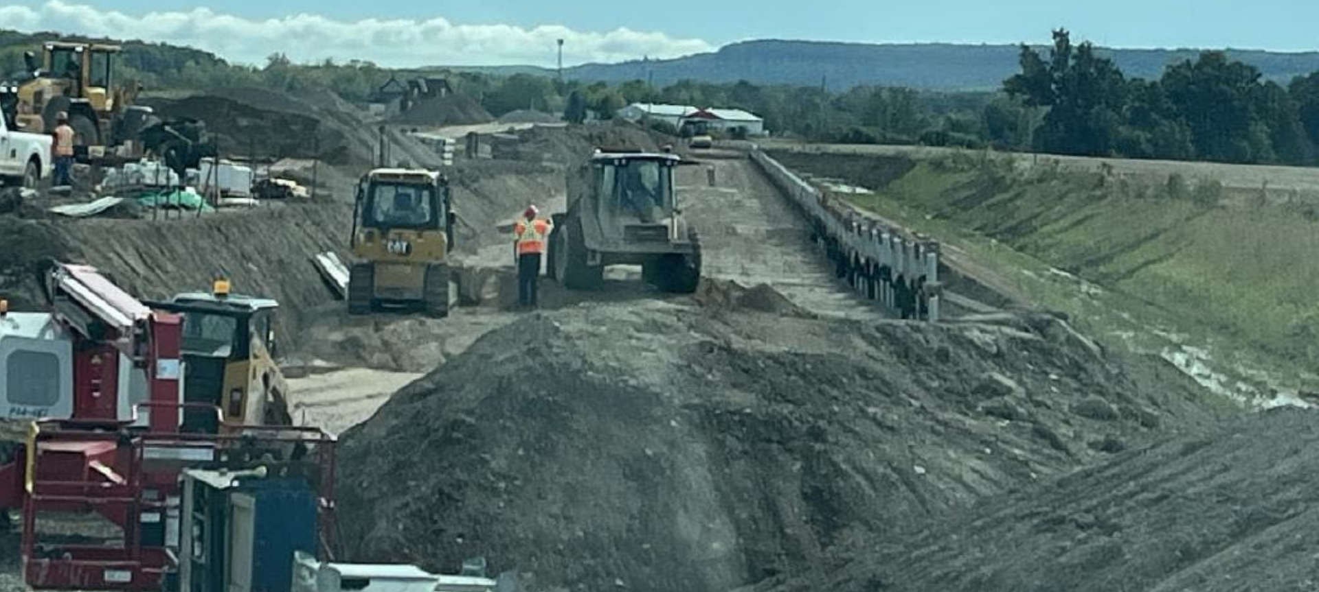
Truck Access Road – Backfilling of material along west RSS wall – Sept. 27, 2024
