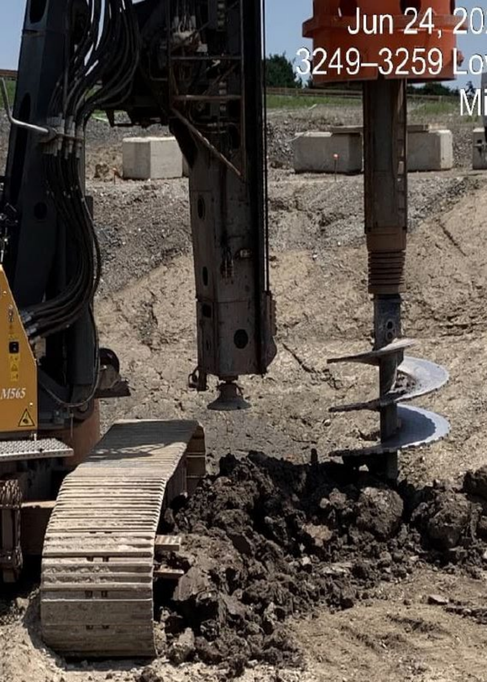
LBL West – Drilling prep and caisson installation for crane pad June 24- July 2, 2024
