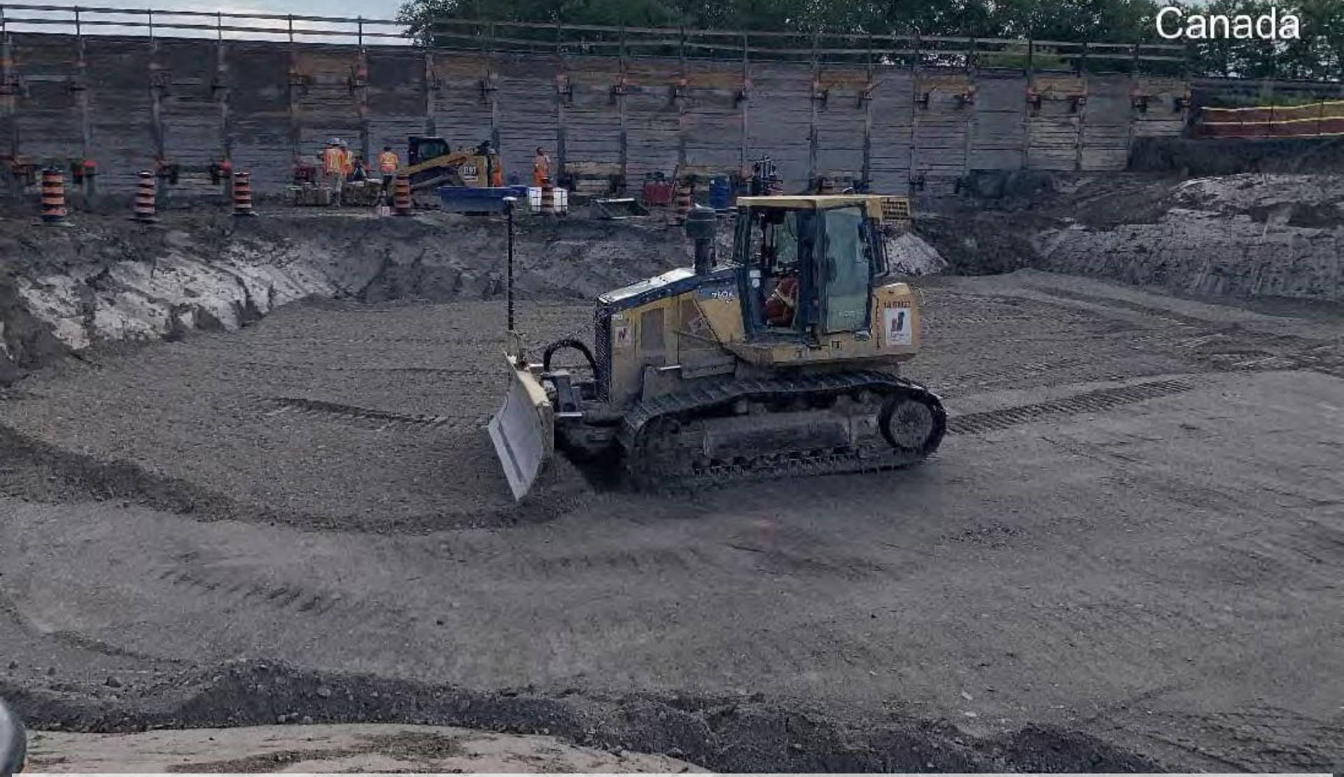
LBL West – Grading prep for crane pad and caissons installation - June 18, 2024
