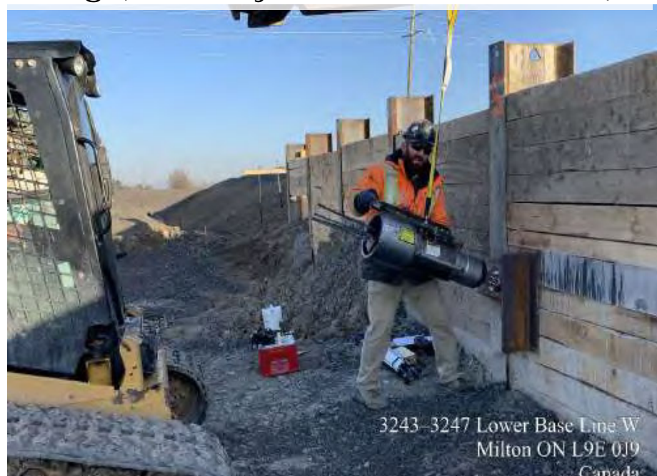
LBL West – Lagging work & Anchor Testing (February 15 to March 1, 2024)
