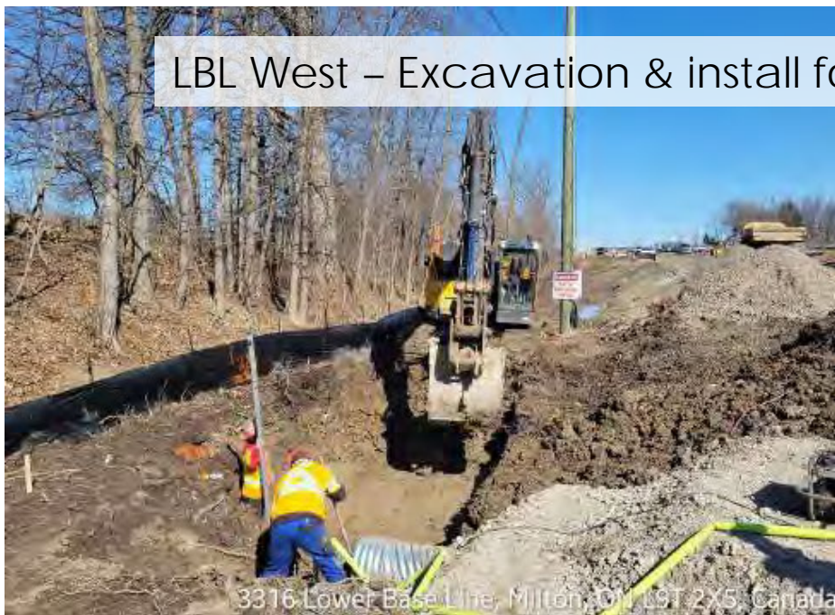
Rip-rap & straw bale install at inlet and backfilling (March 4, 2024)
