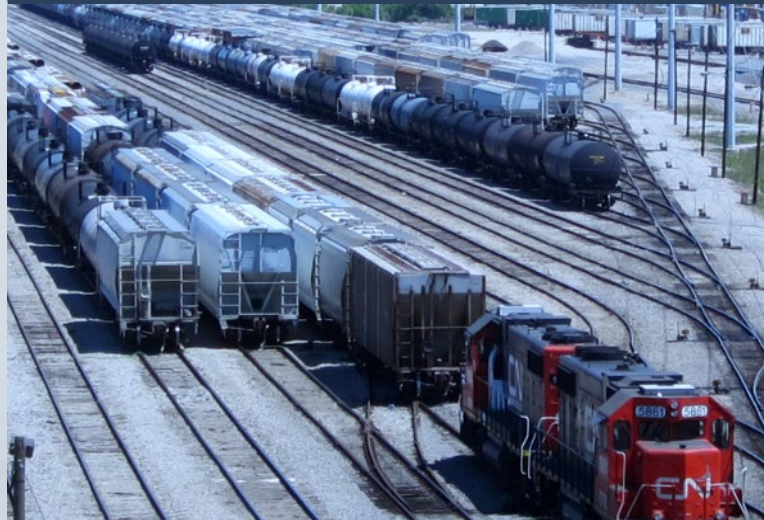
Flat Switching Yards
