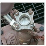
Rupture disc-type pressure relief device
