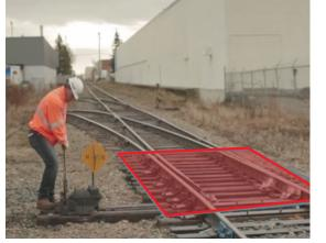
You may have to chip away any ice or snow that prevents the open switch point from closing rightly against the stock rail using the chisel end of the broom. Sweep away any snow and debris from between the open switch point and the stock rail. Always use a broomstick or similar device to remove foreign material.
