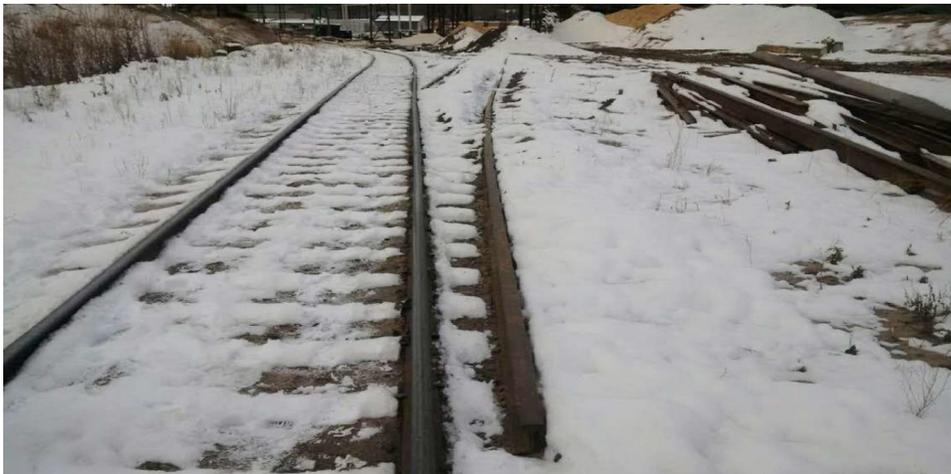
**Flangeways** Be vigilant where flangeways or any trackage might be covered with snow, ice, or other material. Ensure equipment can be operated through flangeway over track.
