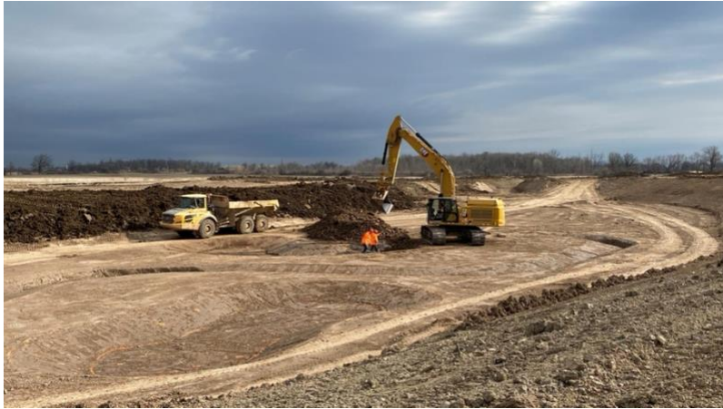
Offline channel construction of Tributary A realignment. April 13, 2022
