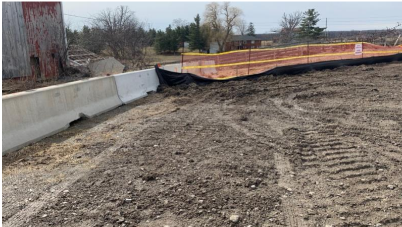
Temporary parking area and heritage barn protection. May 9, 2022
