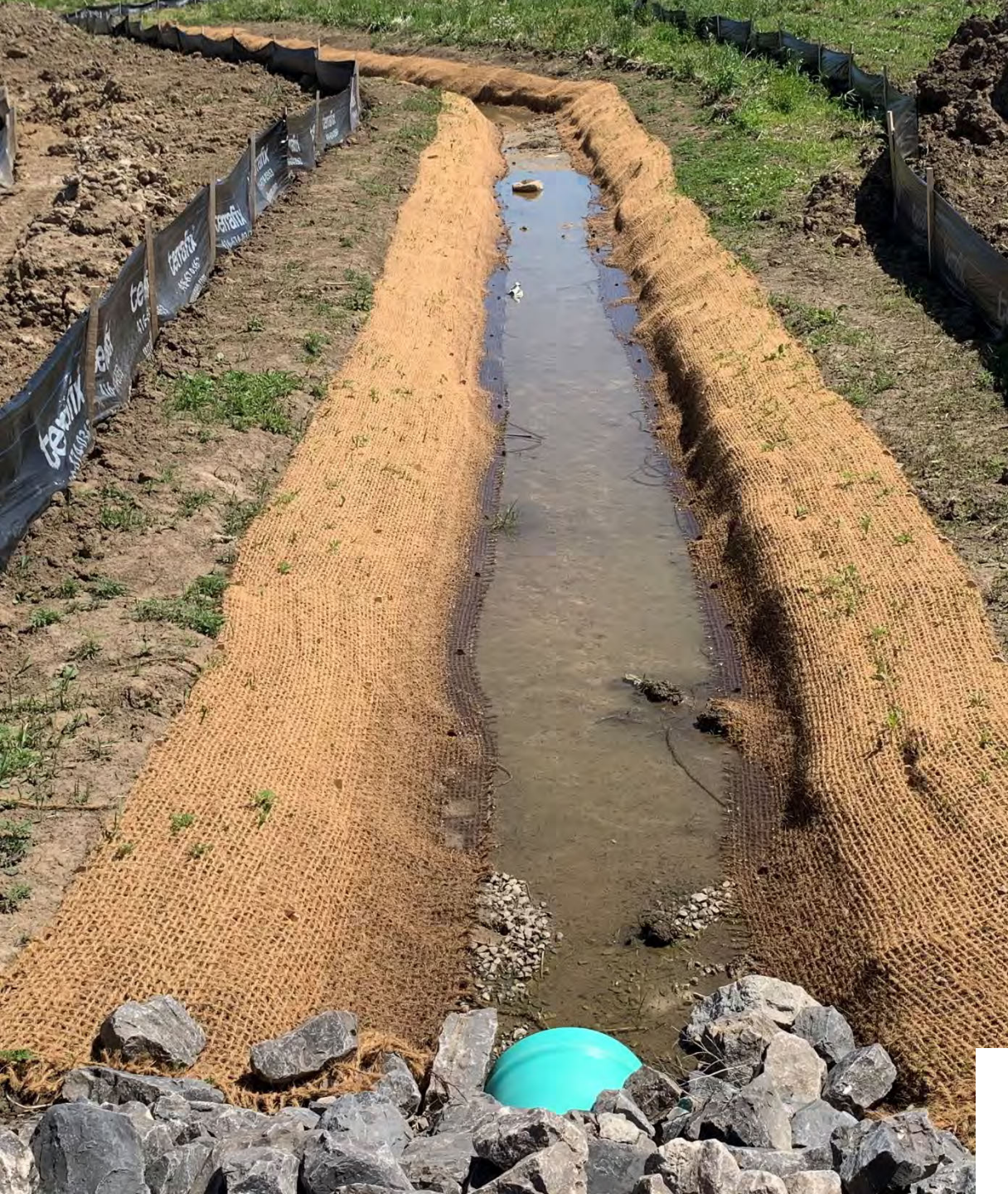
Coir Matting Installed Along Tributary B Stabilizing Channel Banks (June 14 th , 2022)
