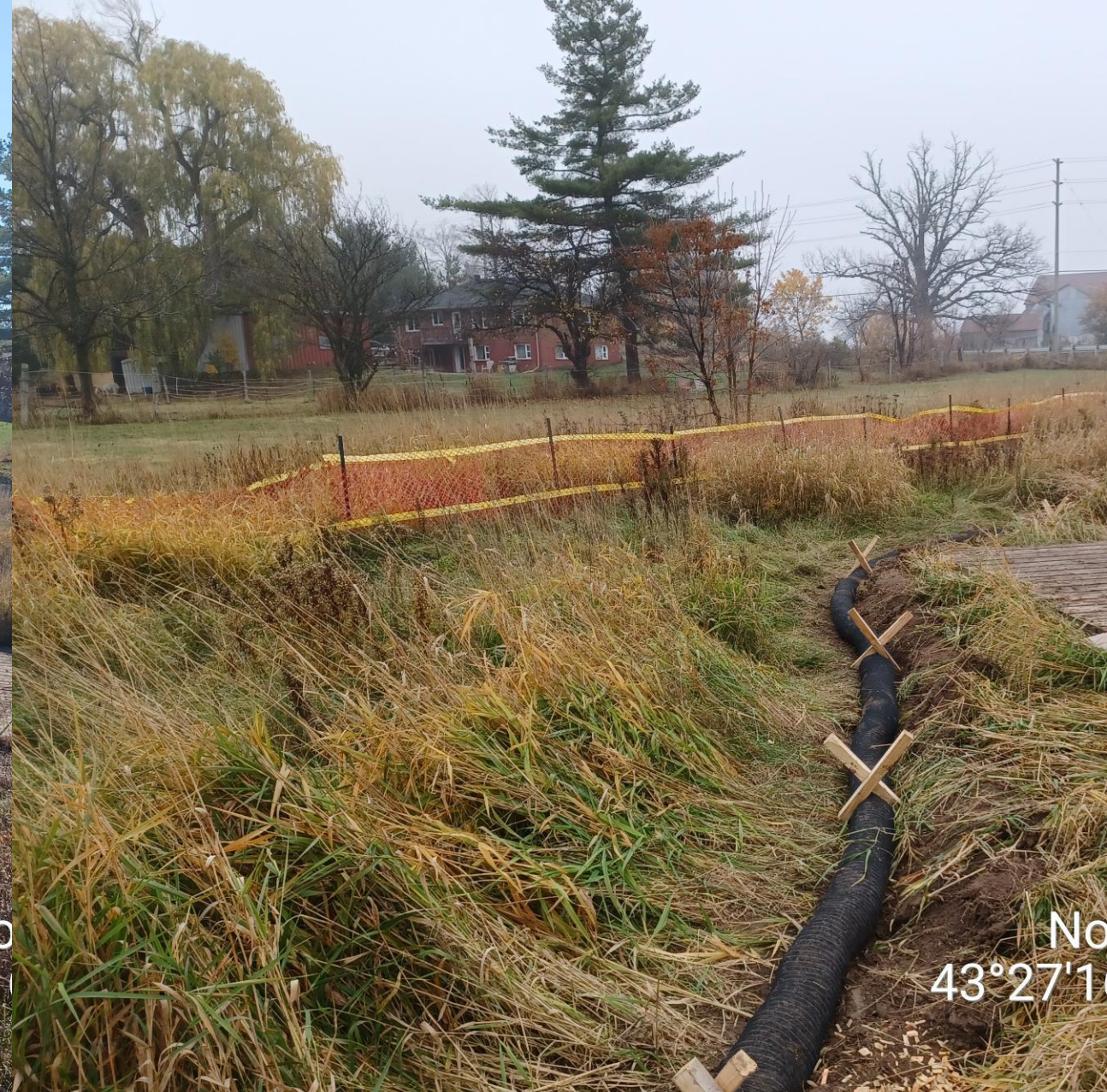
Indian Creek Restoration – Mats and Silt Sock Installation (November 2/3, 2022)
