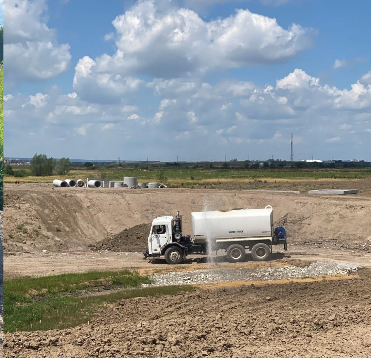
ESCs conditions and dust control measures are permanently monitored on-site (Left: Laydown Area 1 ditch; Right: Dust control on Trib. A realignment). (July 21 st , 2022)
