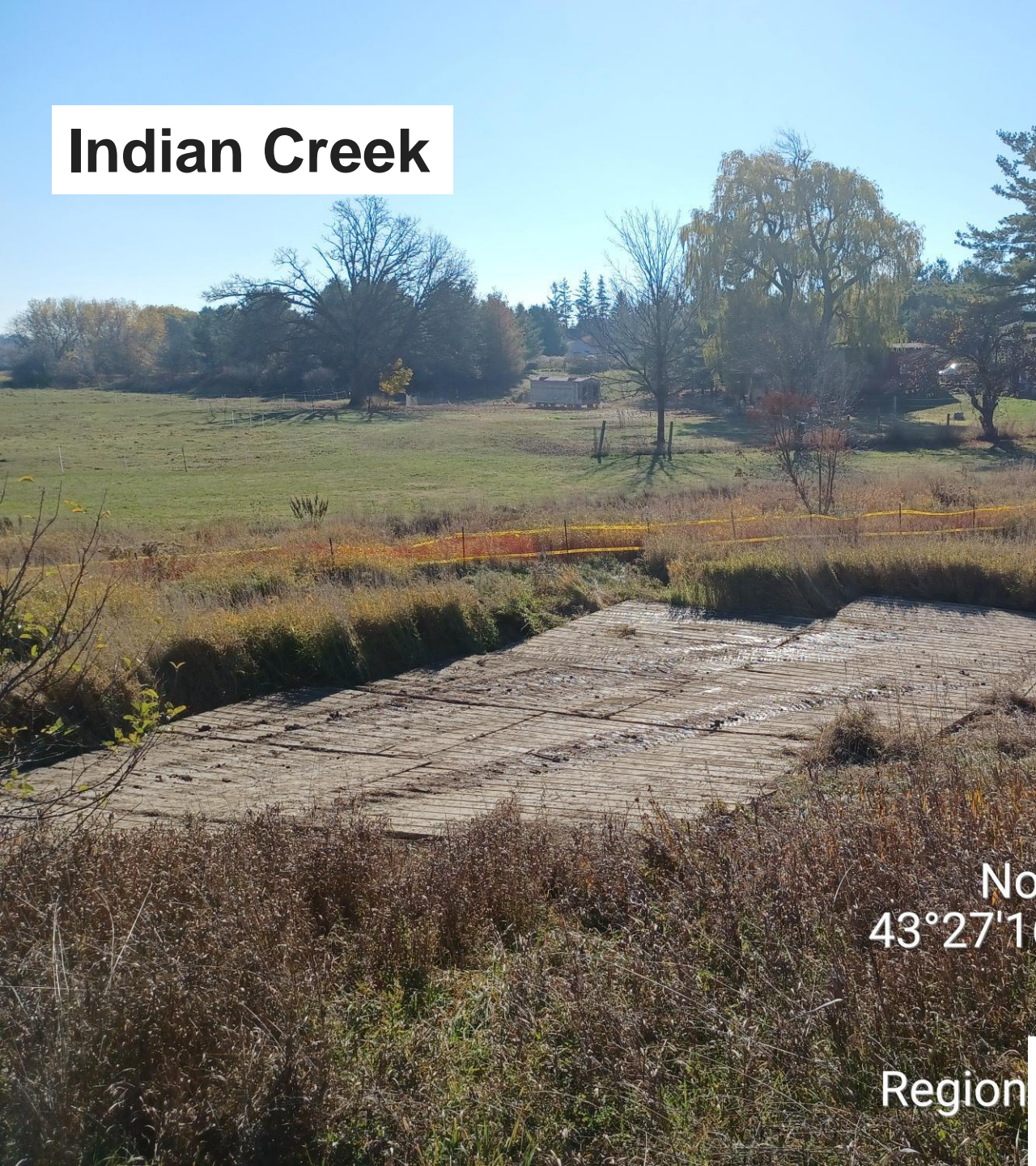
Indian Creek Restoration – Mats and Silt Sock Installation (November 2/3, 2022)
