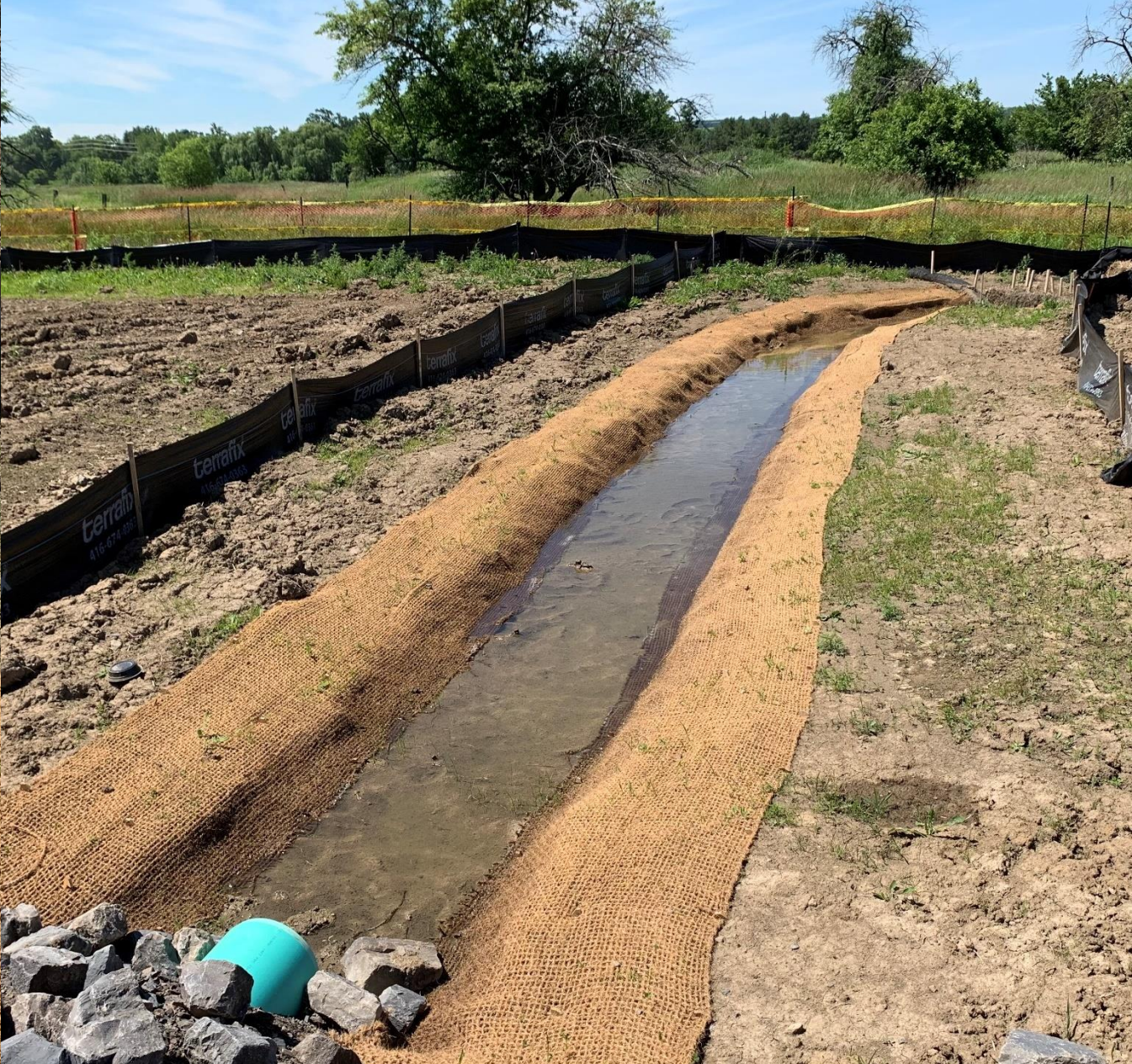
Coir matting at Tributary B stabilizing channel banks. Monitor bed stability and seeding planned for stabilization (June 14 th , 2022)
