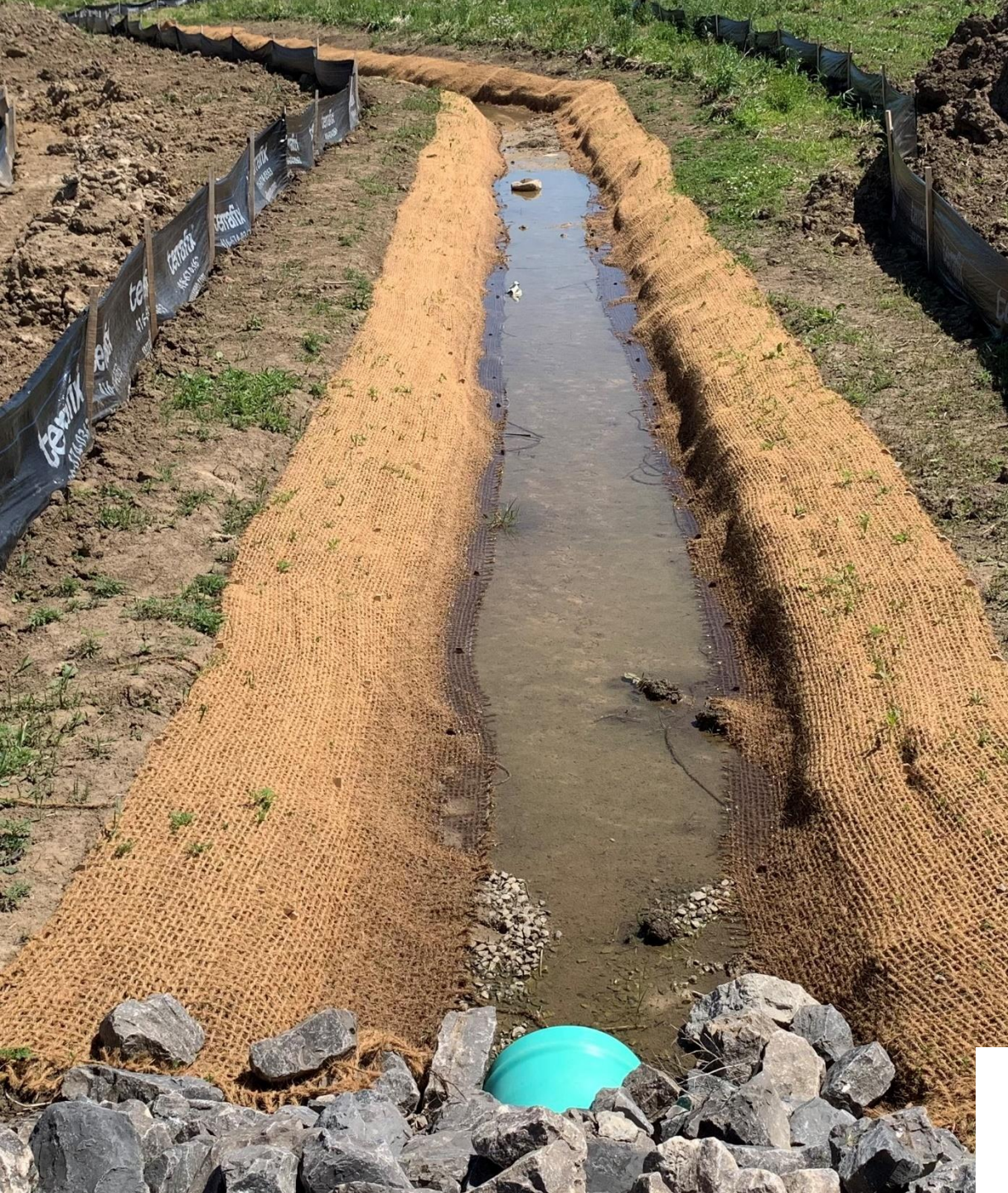
Coir matting at Tributary B stabilizing channel banks. Monitor bed stability and seeding planned for stabilization (June 14 th , 2022)
