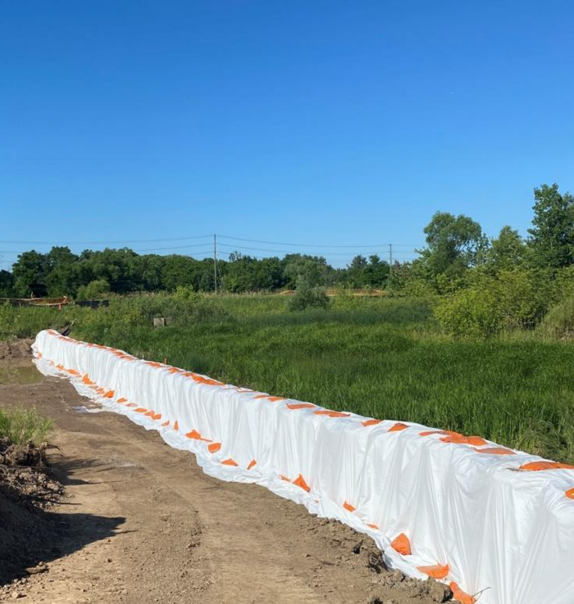
Coffer dam to isolate Trib. A work area from online portion of Trib. A; installed and observed in good standing (July 7 th & 14 th , 2022)
