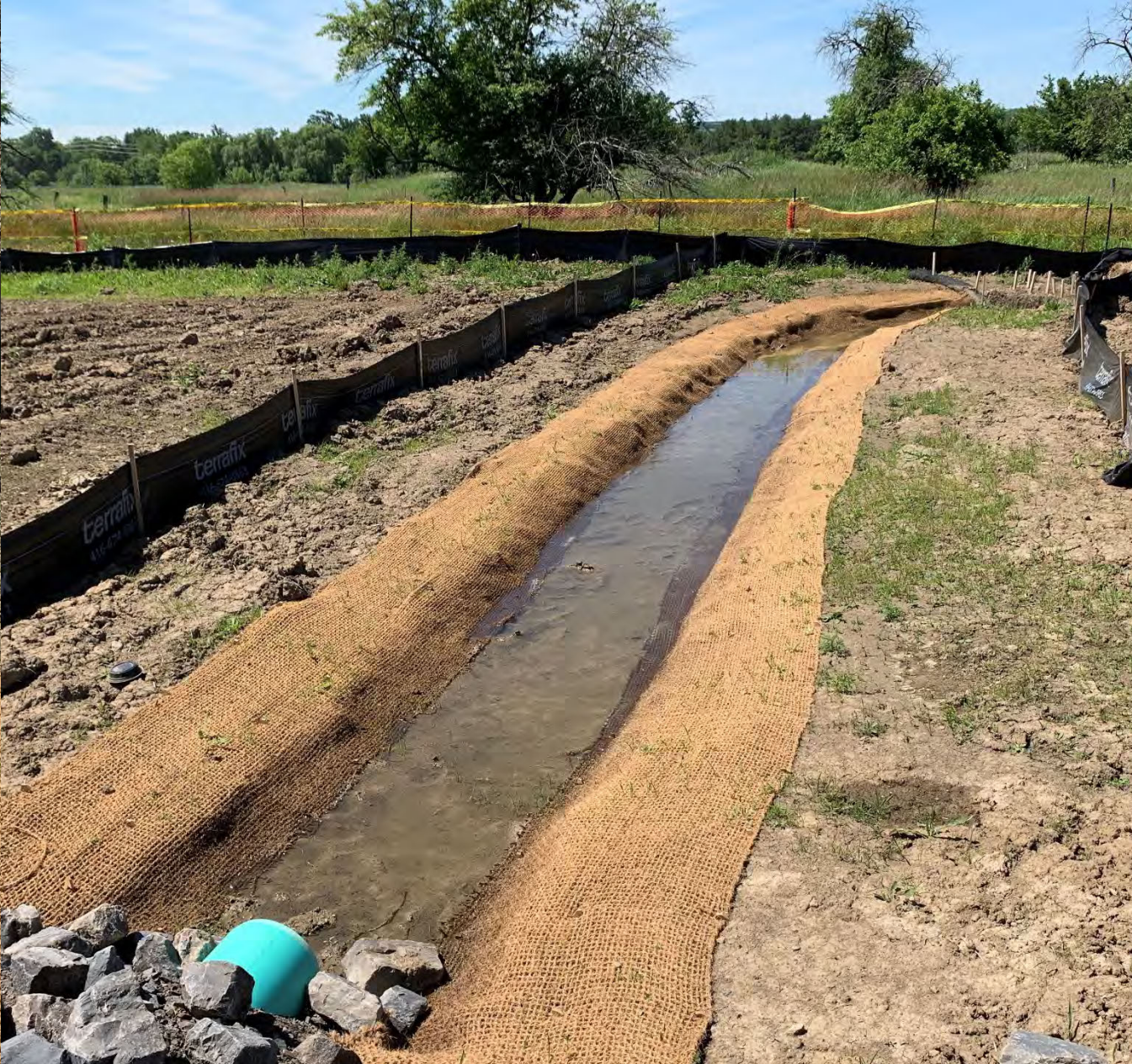
Coir Matting Installed Along Tributary B Stabilizing Channel Banks (June 14 th , 2022)
