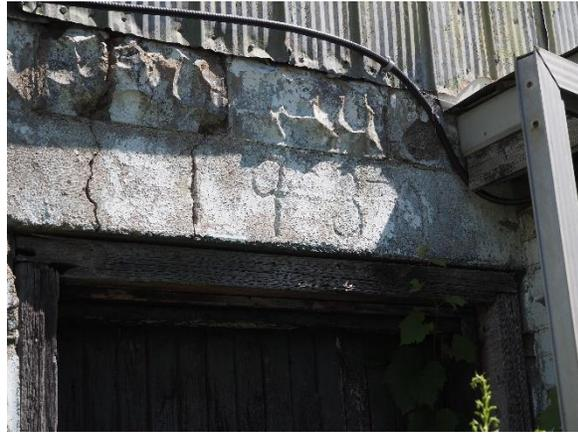
**Plate 42: Cracked lintel above south entrance door**
