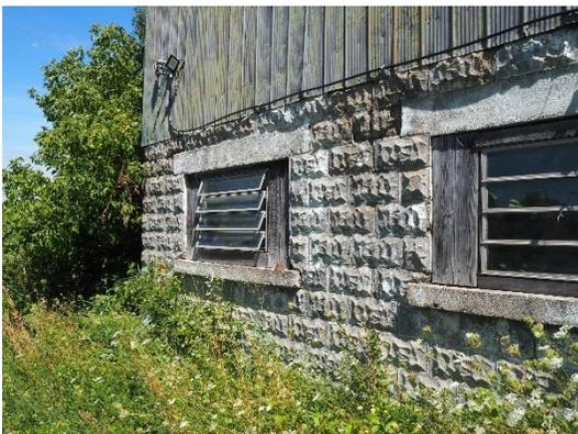
**Plate 22: Rusticated concrete foundation, windows, and metal cladding on south façade, looking northwest**
