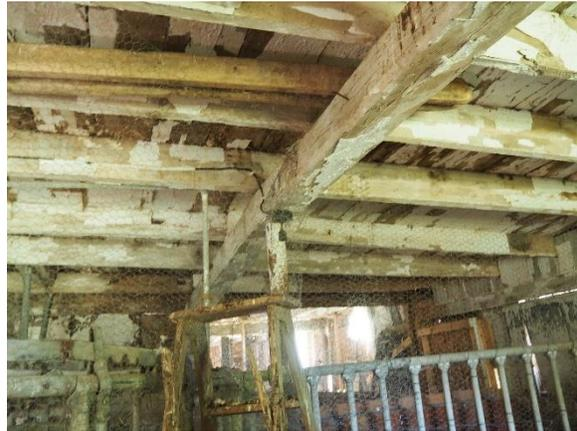
**Plate 29: Hand hewn and machine cut timber**
