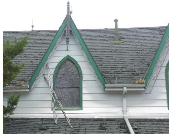
**Plate 29: Worn paint and damaged bargeboard**
