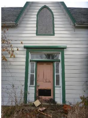
**Plate 2: Front entrance with transom window, side lights and central gable, front façade, looking north**
