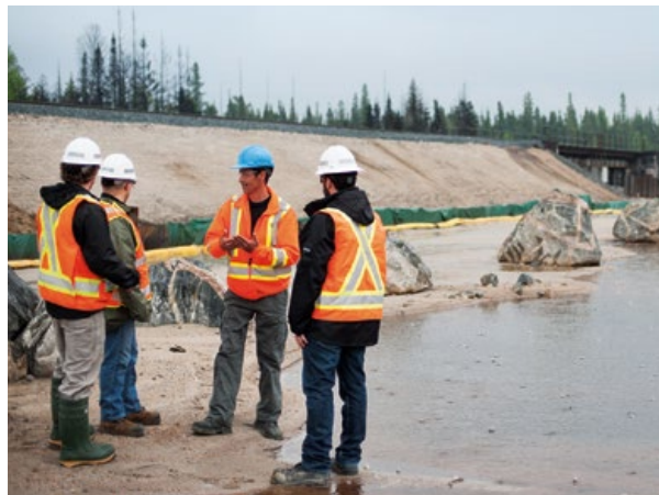
COLLABORATING TO RESTORE GOGAMA: CN and Mattagami First Nation teams are now collaborating on the restoration phase, bringing in clean soil and re-establishing lost vegetation on approximately 10 acres.
