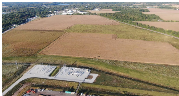
Aerial view looking WSW from Decatur Road – substation in foreground; M-60 Highway on left; CN Rail on right
