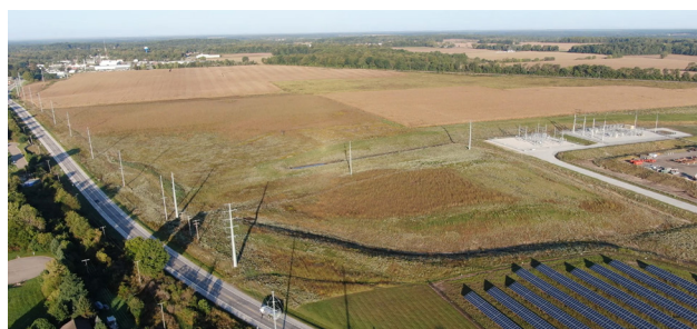
Aerial view looking NW from Decatur Road (south of M-60 Highway)
